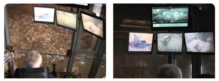
Two FLIR FC-Series R cameras monitor the entire waste storage unit (25 x 25 m).
